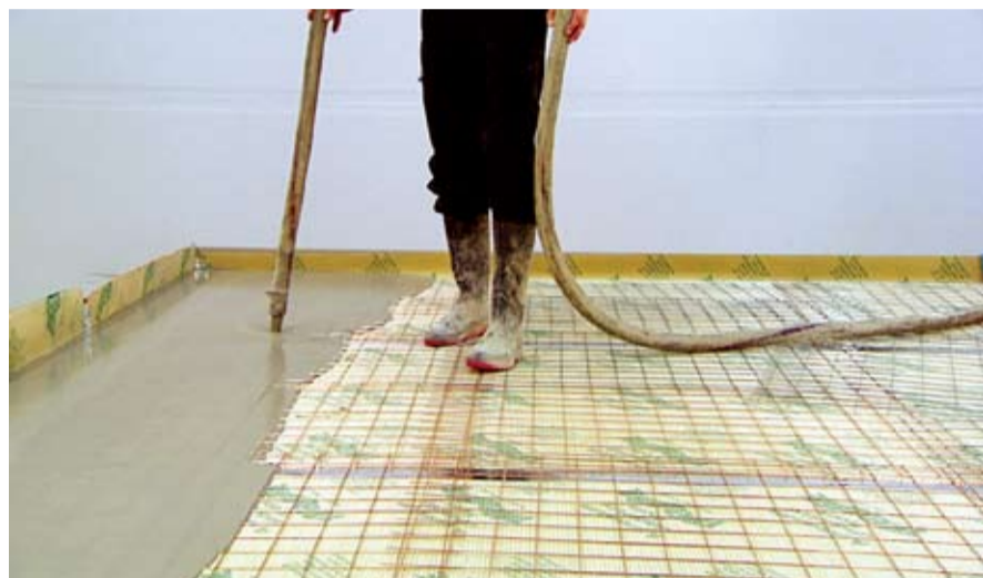
Concrete is poured over the underlay during construction
