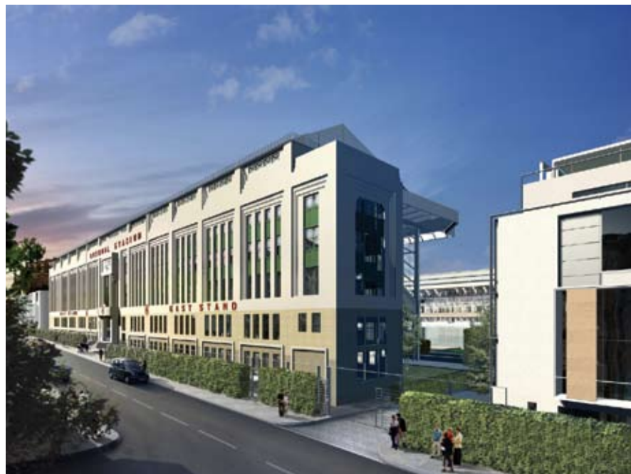
Highbury Stadium Square development
